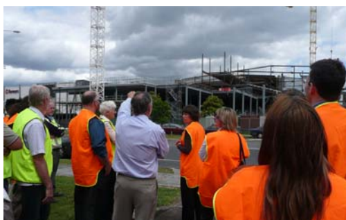
Westfield Manukau Construction Site
