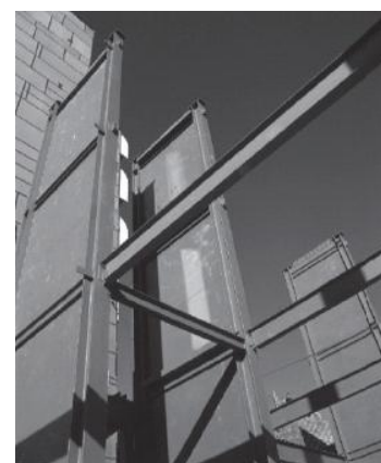
Steel Plate Shear walls
