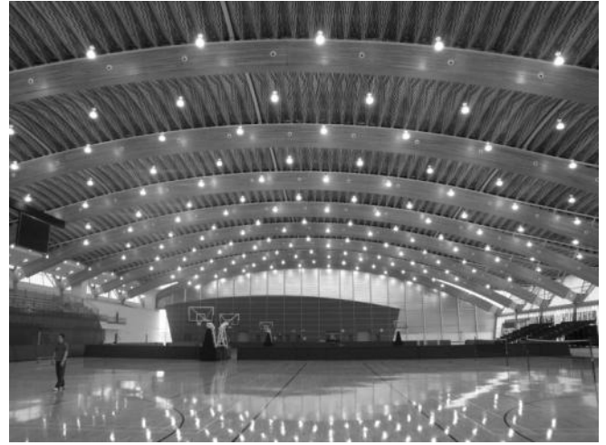
Vancouver Olympic Speed Skating Oval, featuring composite steel/timber trusses.
