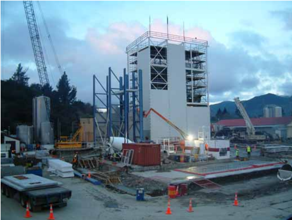
Making good progress four weeks later
