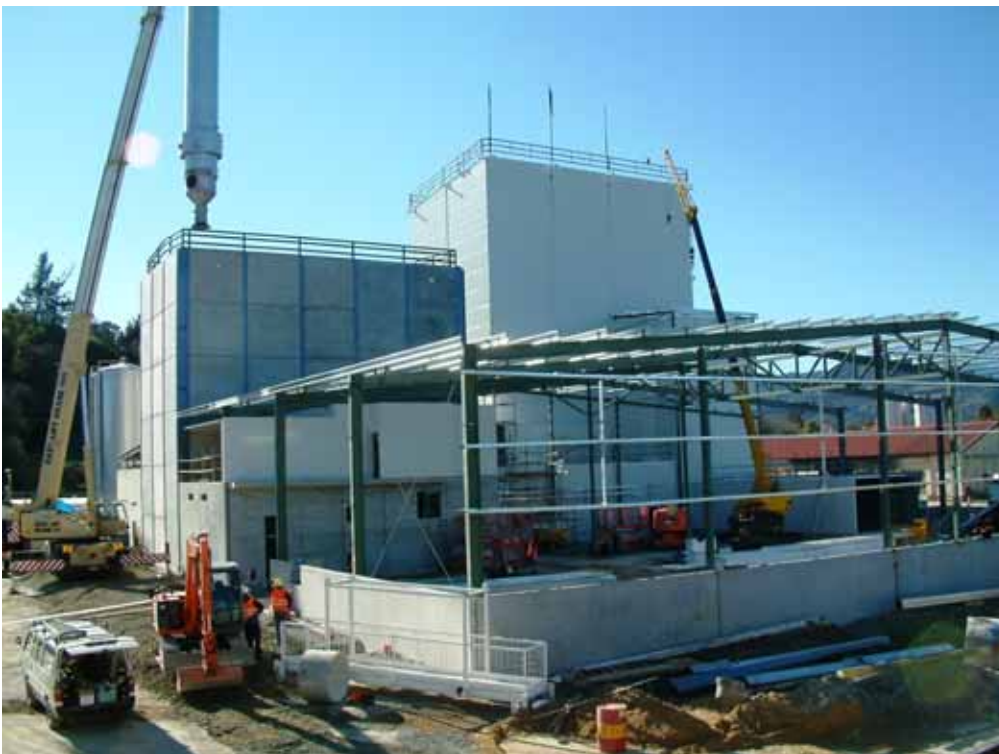
The Takaka Dairy Plant, close to being reinstated
