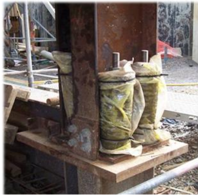
Rocking detail featuring Ringfeder springs.
