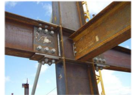
Sliding hinge joint.
