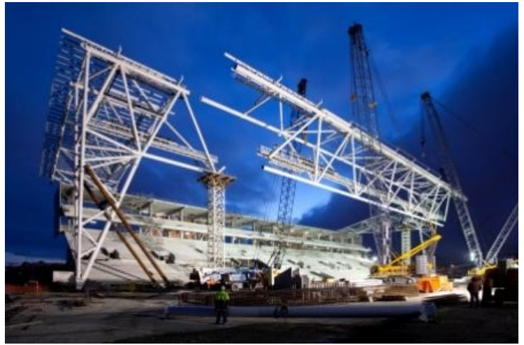
Construction in progress on the Forsyth Barr Stadium.
