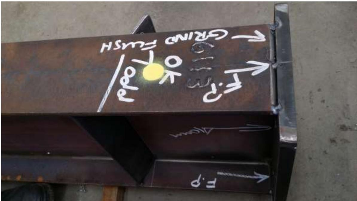
**Figure 3: Inspected and approved weld preparation**
