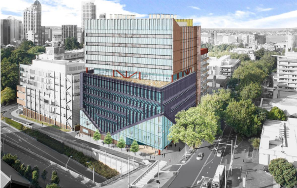
In 2010 the University of Auckland embarked on a five-year project to upgrade its Faculty of Science buildings. The \$290 million redevelopment consisted of the refurbishment and seismic strengthening of two existing buildings, construction of a new link structure, and demolition of two buildings to make way for the new Science Centre Tower.
