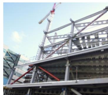
Given the high degree of seismic engineering involved, precision and verification were critical. Multiple grades of steel were employed on the job and each required a certificate of authenticity; independent weld inspections were carried out by a third party; and in the interests of transparency, and in line with all projects completed by a New Zealand fabricator, a quality manual was produced for the project. Product traceability is assured.
