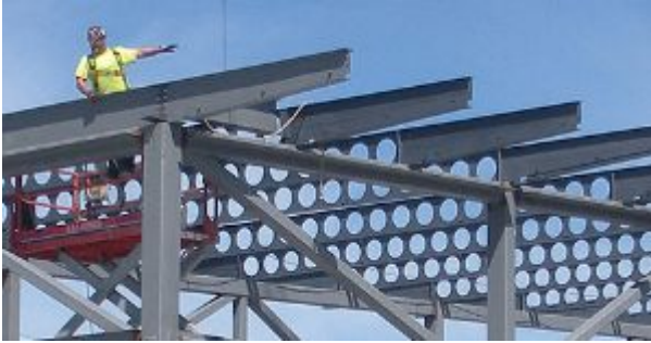
Welded beams being used in construction
