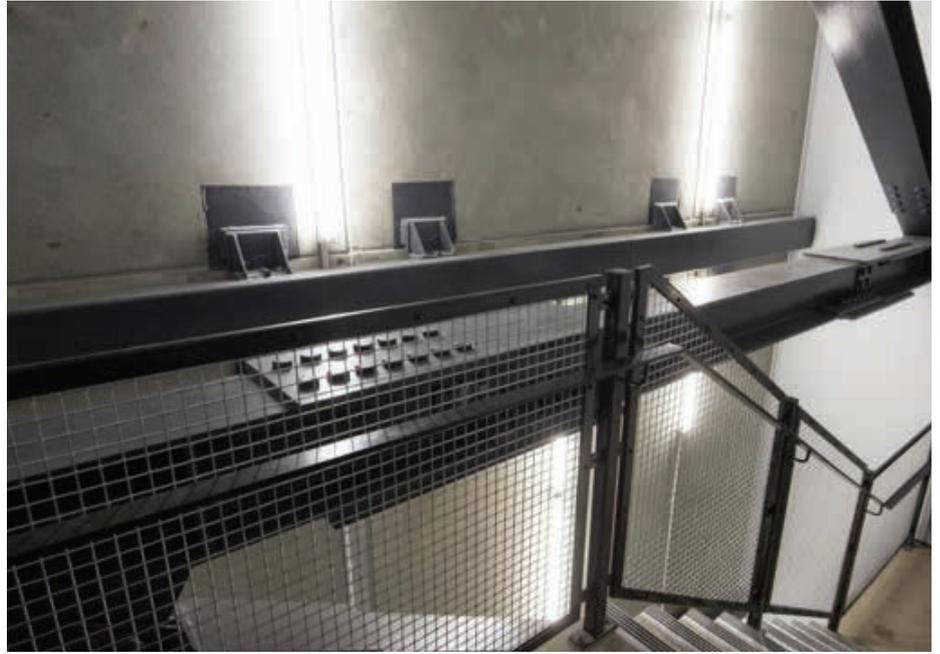
Designed after the Christchurch earthquakes, Te Piringa's seismic preparedness was considered – and it's impressive. Even when exposed to large earthquakes, the steel absorbs seismic forces beam to beam due to their rotation capacity. This system is an alternative in New Zealand and a proprietary product, with just a few global suppliers.
