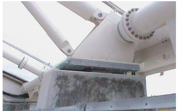
Figure 7: Bearing at north end of an ETFE transom
