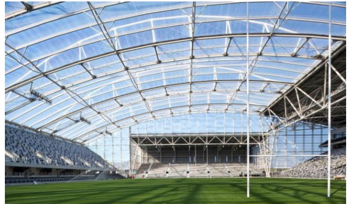
Figure 4: Roof structure with East Stand beyond
