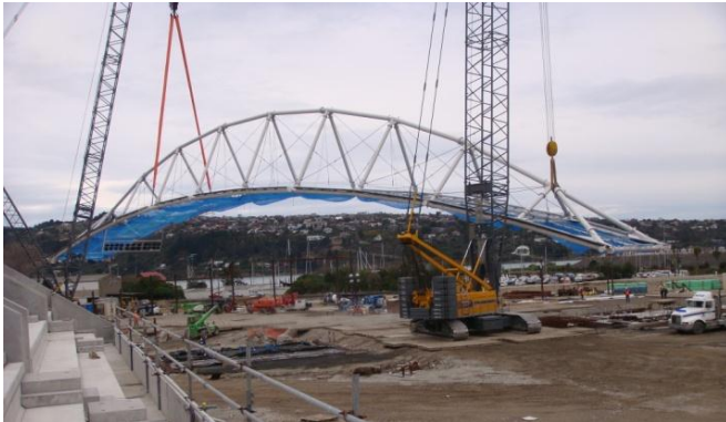
Figure 6: Arch truss being maneuvered across the site
