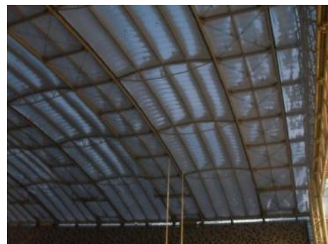
Figure 10: Roof under light snow load
