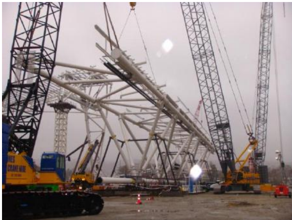
Figure 13: Primary Truss assembly
