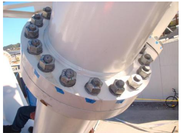
Figure 11: Typical flange joint
