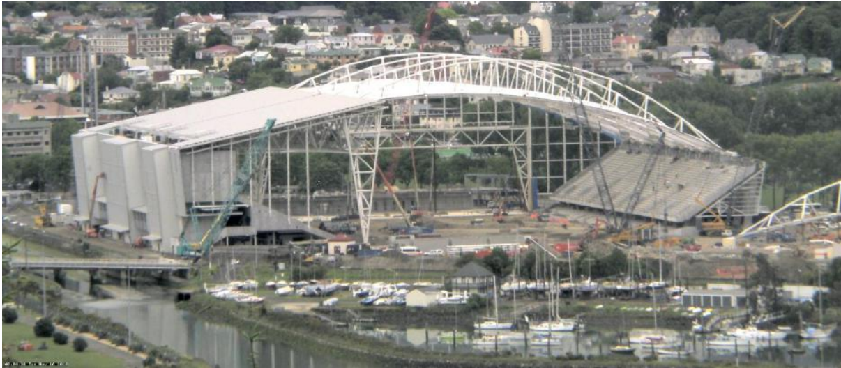
Figure 1: Under Construction - 16 Nov 2010
