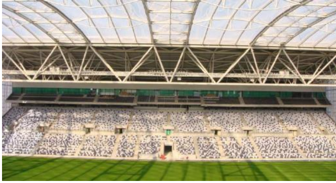
Figure 2: Main Roof, Primary Truss and South Stand
