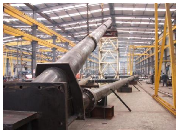
Figure 12: Trial assembly of Primary Truss leg
