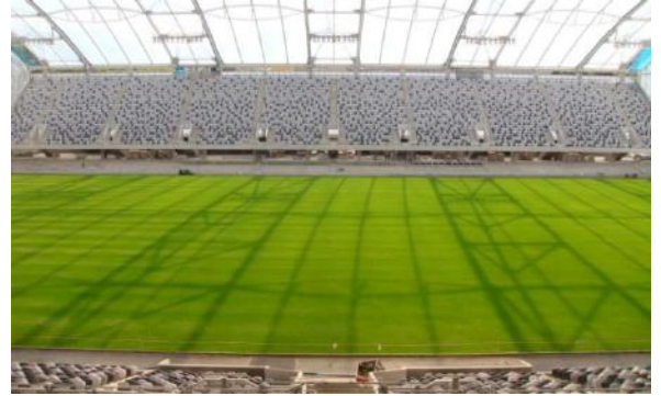
Figure 3: Main roof structure and North Stand
