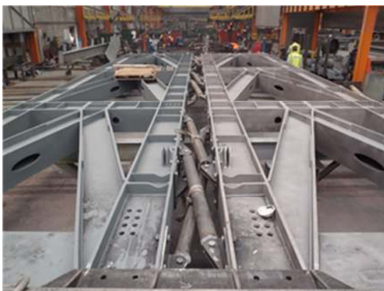
Figure 5: Pair of steel braced frames assembled in the workshop with dampers
