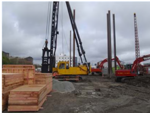
Figure 13: Steel H-piles being driven to approximately 24m
