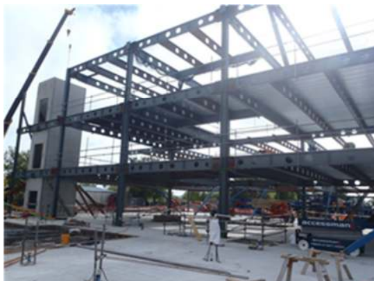
Figure 11: Concrete-steel composite floor structure under construction
