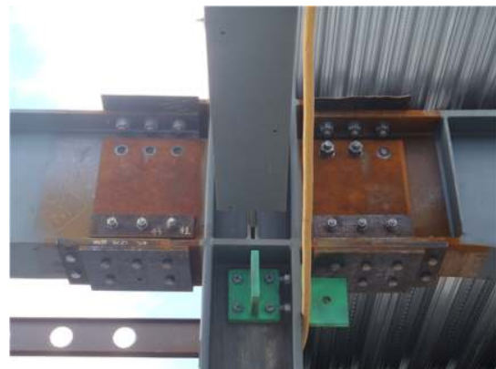
Figure 12: Sliding Hinge Joint for secondary frames during construction
