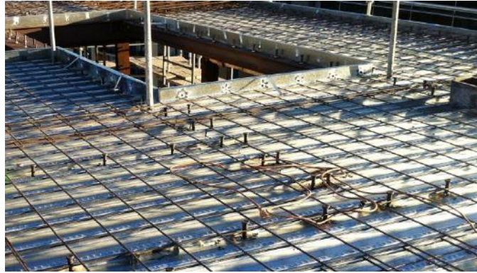
Figure 1. Composite slab in a steel frame structure.
