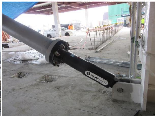
**Figure 9:** Frame with the viscous dampers in place
