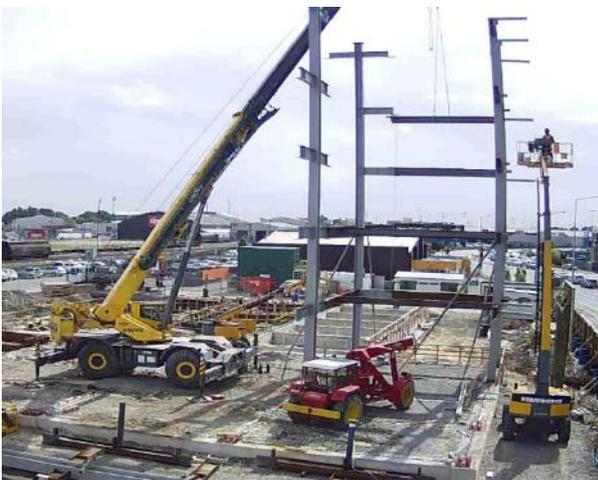
**Figure 8:** Erection of columns
