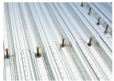
Figure 5. Butt joint in decking (correct positioning of single stud per trough)
