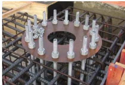
Figure 7: 3D SAP2000 model (CSI, 2014) of column base connection showing bolts in tension (left image) and a site photograph with the base plate and HD bolts in place (right image)
