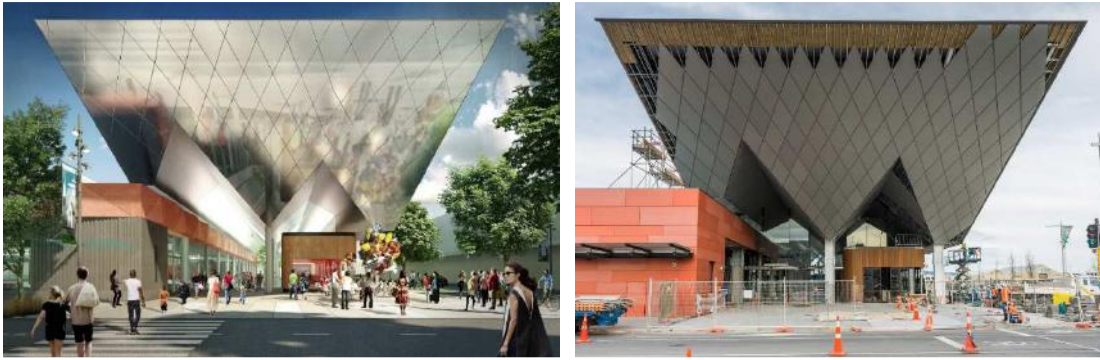
Figure 4: Architect's impression of the Christchurch Bus Interchange: Main Entrance Corner Cantilever and photograph of Bus interchange under construction, right image (image courtesy of Architectus)
