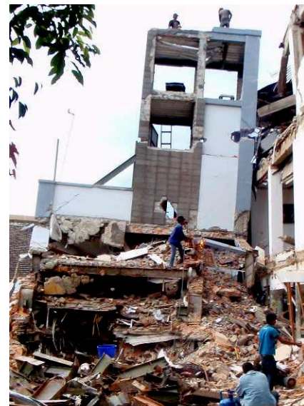
Figure 4: Steel MRF Weak Axis Collapse of 5 Storey
