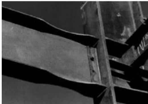
**Figure 1: Reduced Beam Section Moment Connection (Englehardt et al, 1996)**
